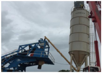
The installation of the mobile concrete plant MobKing-60, sent to the Republic of Mali along with its spare parts, has been completed in the city of Sikasso. The machine was installed on-site by CONMACH mechanics. The mobile concrete batching plant with a 4 x 10 m³ bunker, with a capacity of 60 m3 / h, has a 1 m³ concrete mixing capacity. The installation of concrete batching plant with a single-shaft mixer was completed after the installation of a 75-ton cement silo.
